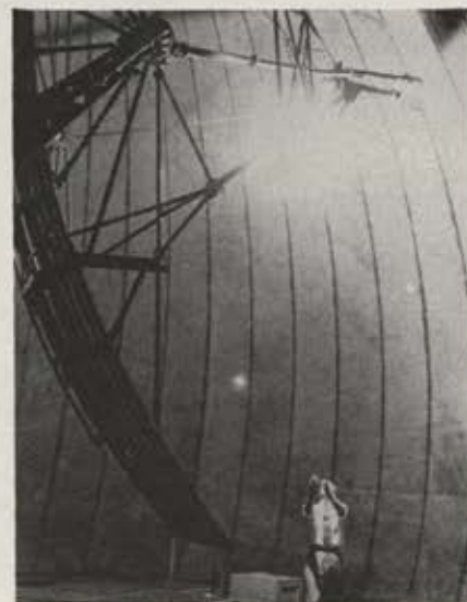
A flashbulb ignited in mid-air by the energy radiated from a powerful new radar provides light for this photo.
