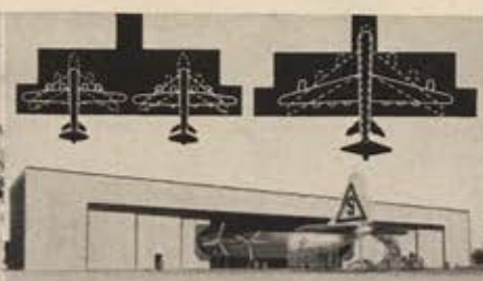
ALL-PURPOSE "WING" HANGAR accommodates one heavy aircraft or two medium aircraft.
