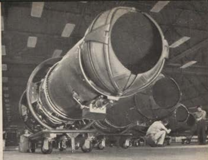
AUTOMATIC CONTROL of the variable area nozzle (illustrated above) regulates exhaust velocity and temperature.
