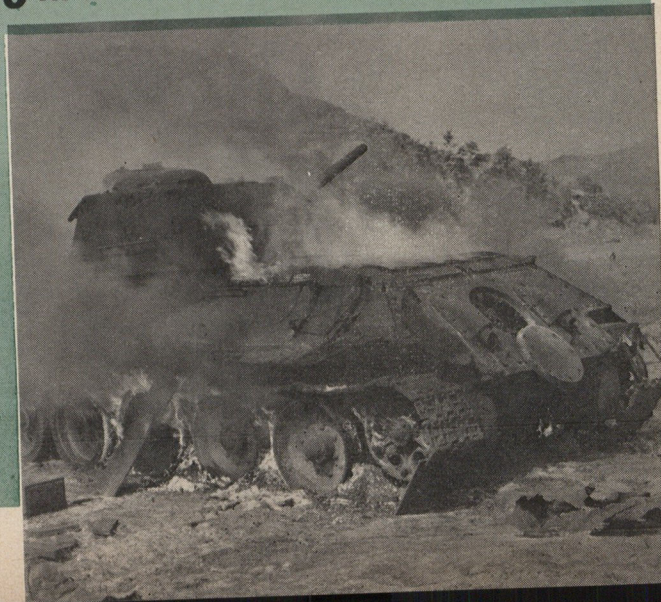
5 Closeup of smoldering T-34 as scene clears. Except for the rear wheel, everything combustible has burned.
