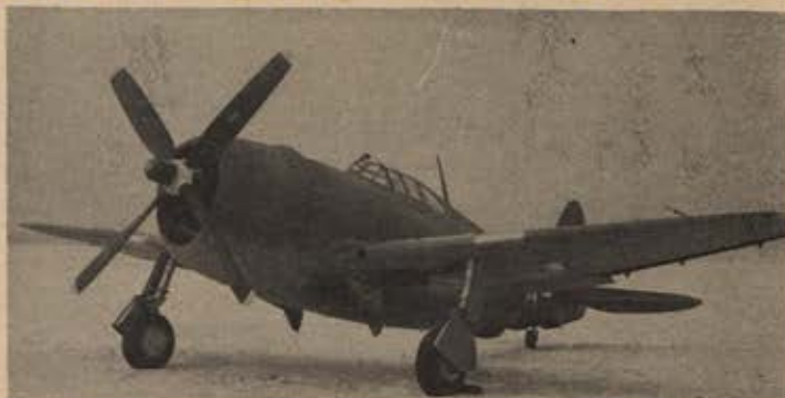
The only E built was an experiment with sealed pressure cabin.
