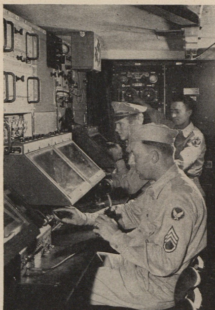
Radar-operated Ground Control of Approach system is housed in trailer unit shown above. Interior view, below, shows operators directing incoming plane onto correct flight path.
