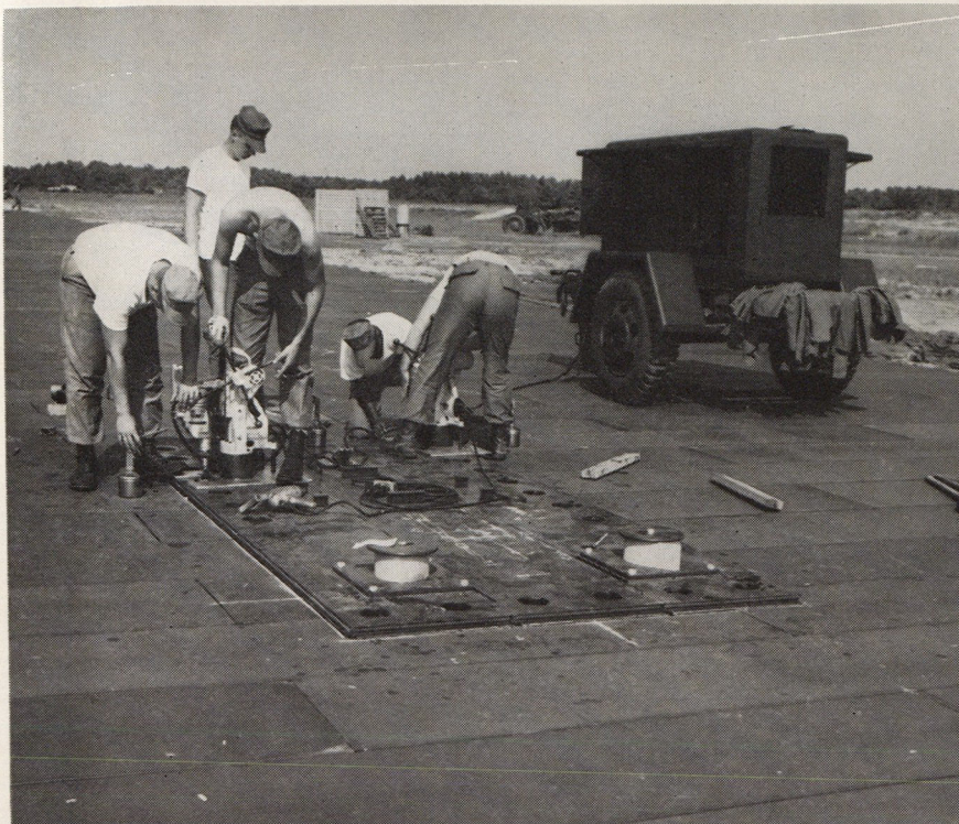
As the new runway nears completion, Marine launch and recovery technicians install the dolly-arrester assembly. Nylon rope is reeved through the sheaves on this assembly and on an identical assembly at the other end of the runway to stop the catapult dolly.
