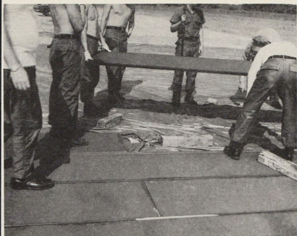
Members of naval construction battalion, "Seabees," begin laying the aluminum mats that, when finished, will make up the SATS runway 72 feet (21 m) wide and a little more than 2,000 feet (610 m) long. Sections hook onto each other.
