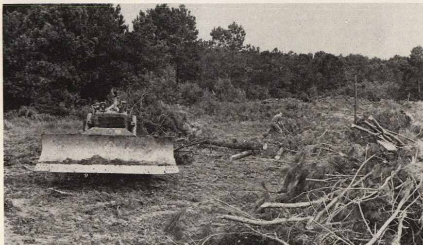
Airfield in the making—Marine Corps engineers clear away trees and underbrush for construction of the world's first SATS operational training site, Bogue Field, N. C.
