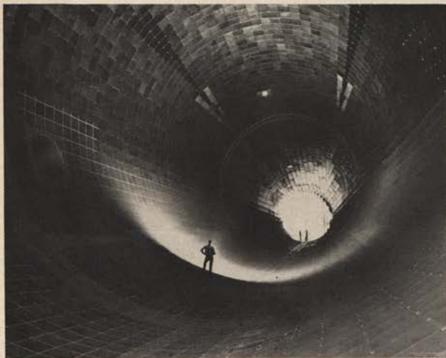
Dimensions of one section of new supersonic propulsion wind tunnel being built at Arnold Engineering Development Center, Tullahoma, Tenn., are illustrated by size of technicians checking its interior. It is lined with stainless steel to handle the 650° F airflow needed to simulate flight velocities up to Mach 4.
