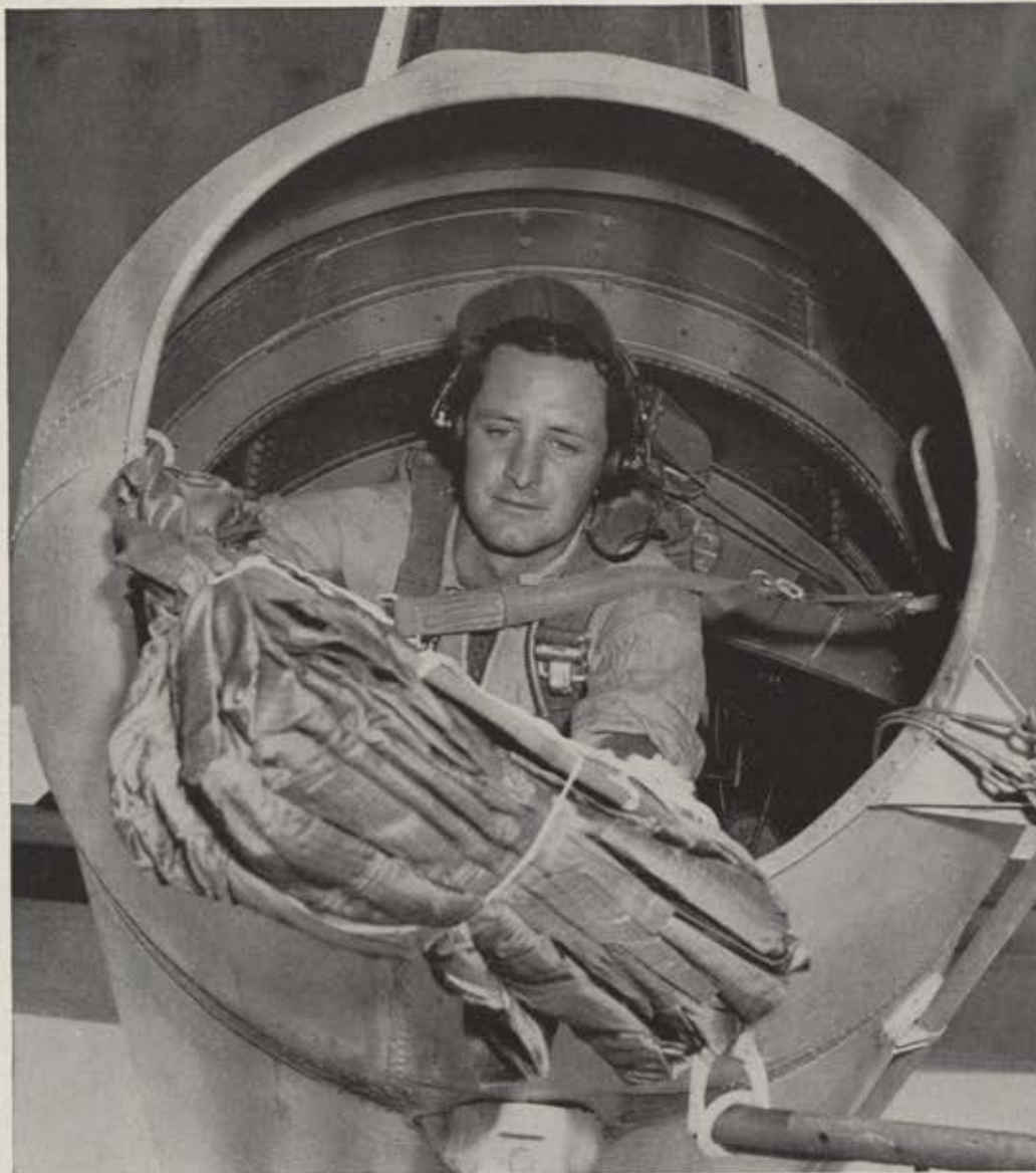
▲ A/IC Richard B. Landreau shows how to launch a sleeve target from a B-29. The metal rod (lower right), called a "fish," releases targets not shot away.
