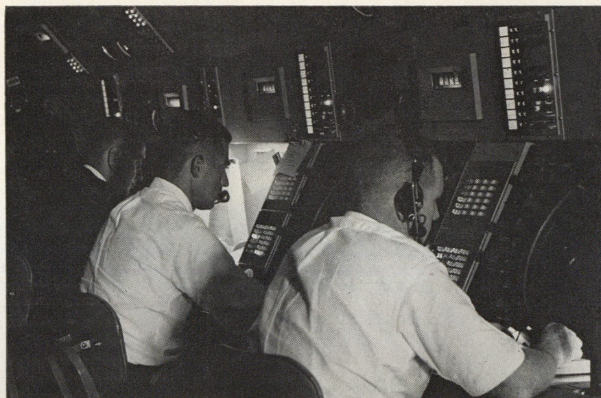
Busy FAA airport control towers are equipped with both precision-approach and surveillance radars. Shown here at Dulles International Airport is one of the newer installations. The radar, and radio, are used to keep tight control over traffic, making all flying safe.
