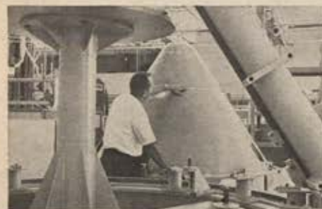
The outer shell. The other main part of the command module is a heat-proof stainless steel honeycomb shield which fits over crew compartment. The two shells join early in the fabrication process for an exacting compatibility test. This remarkable stainless steel honeycomb technology was first developed by NAA for the XB-70.
