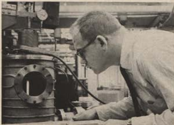
1st Lt. Nathan G. Tupper, a 1962 Air Force Academy graduate, is a metallurgical engineer working, above, on creep-testing of a refractory metal at the Division's Materials Laboratory at Wright-Patterson.
