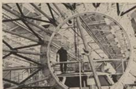
Precision jig. Shaping one Apollo crew compartment requires seventy giant tooling jigs similar to this one. Each jig is built to exact measurements, optically checked. This is why North American Aviation fabricators can hold to tolerances as minute as .010 inch on a space vehicle that stands 14 feet high, with a 13-foot base diameter.
