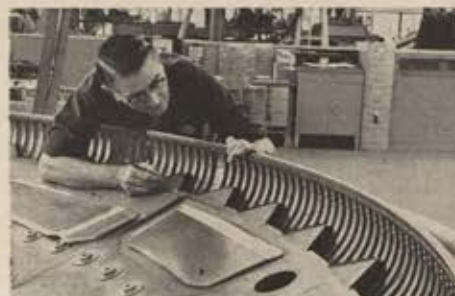
Heat shield. Bolted to bottom of inner crew compartment, this shield must bear re-entry temperatures as high as 5,000°F. The outer shell then leaves NAA to be covered with the ablative heat shield. Ablative material is held in a fiberglass honeycomb matrix providing positive attachment method to assure high thermal-structure reliability.
