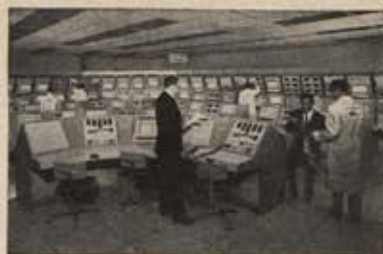
ACE S/C Control Room
