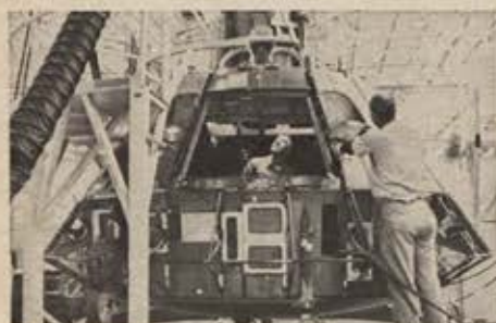
The inner shell. At NAA/Space & Information Systems Division, the inner crew compartment of an Apollo command module takes shape. This leak-proof, pressure-tight shell is made of 2014 T6 alloy, 40% stronger and lighter than commonly welded aluminum alloys. To weld this structure, NAA made epic advances in tooling technology.
