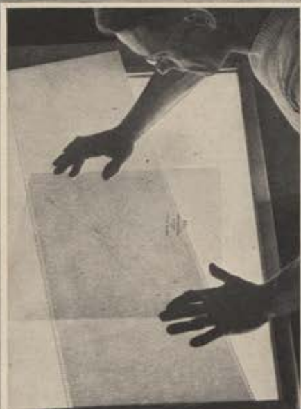
Chart, which can be read to .0005 accuracy, is checked against master pattern on a transparent template.
