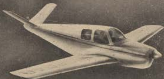
Model 35 The new Beechcraft Bonanza cruises at 175 mph., consumes 10 gallons per hour, carries four 170-pound people and 100 pounds of baggage, lands at 46 mph. Its range is 750 miles at 165 mph. It has a direct operating cost of as low as 1 cent per passenger mile. It's delivered complete for day, night and instrument flight.
