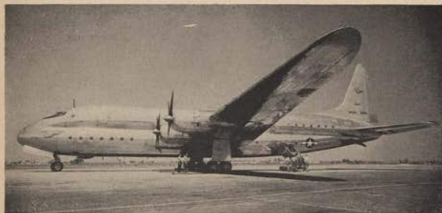
Largest plane ever acquired by Navy, Lockheed's 92-ton Constitution has 189-foot wingspan.
