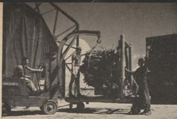
At the Tear-down Shop, parts were removed from used engines that were being sent to the United States for fourth echelon repair. All other maintenance was accomplished on Saipan.
