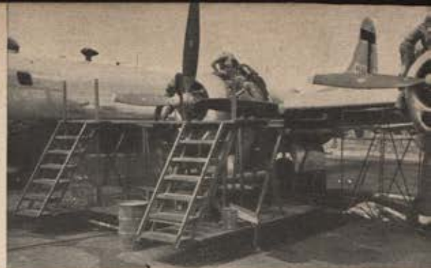
First called "the Monstrosity," this crew stand was later made in the States on specifications of the sergeants who built it with parts of a sugar mill.
