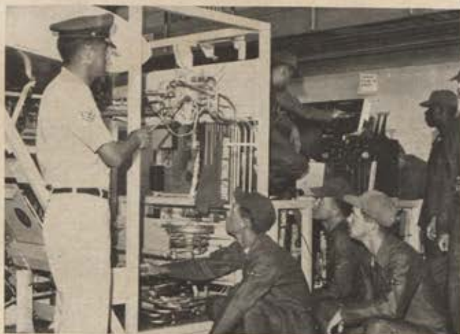
The workings of the complete elevator, stabilizer, and rudder control and trim systems are being studied by these students of the basic jet aircraft course at the Sheppard AFB, Tex., Department of Aircraft Maintenance Training. Mockup is used to show students working parts of systems.
