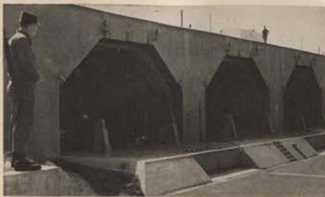
Hardened sites for the Mace-B surface-to-surface tactical missiles became operational during the year at USAFE's Bitburg AB Germany. The sites provide increased survivability for the Mace-B missiles assigned to USAFE's 71st Tactical Missile Squadron, part of 38th Tactical Missile Wing.
