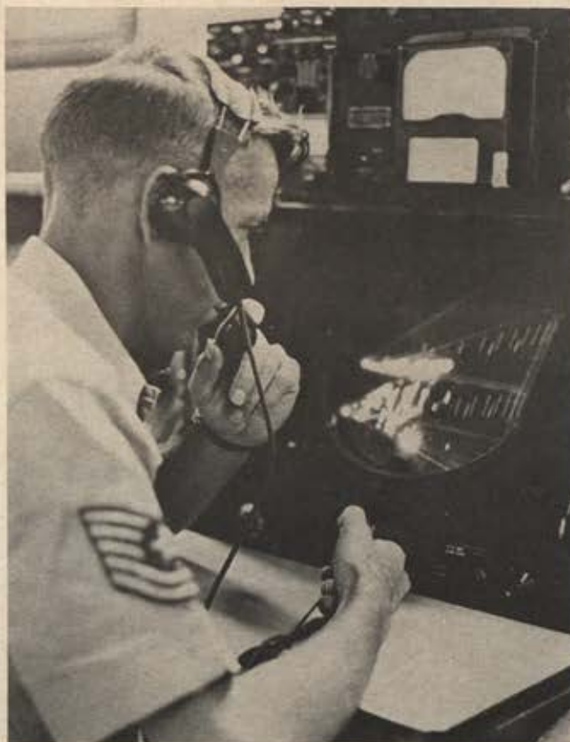
Guiding aircraft to safe landing, whatever the weather, is the job of this RAPCON (radar approach control) technician, another of varied functions performed by AFCS.
