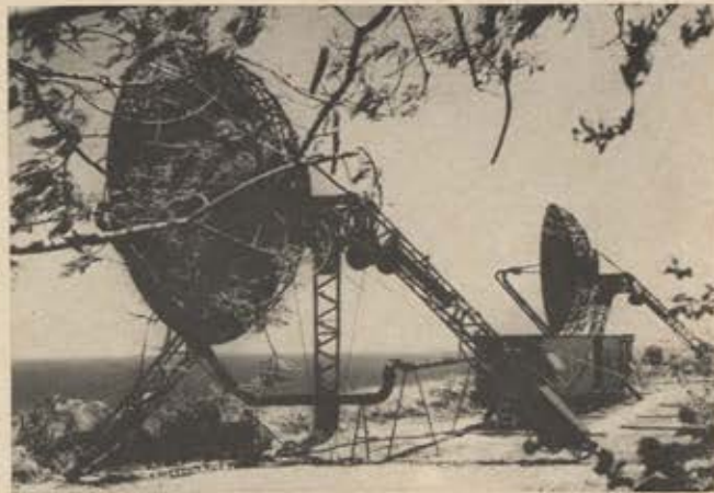
This mobile tropospheric-scatter unit was set up in Puerto Rico in May by AFCS and Bendix technicians to provide communications link with US forces sent to Santo Domingo.
