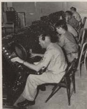
The technically skilled airman requirement continues to be critical, pyramids training costs, often restricts Air Force project continuity.
