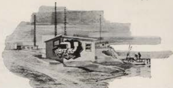
Paralleled primary mobile power
