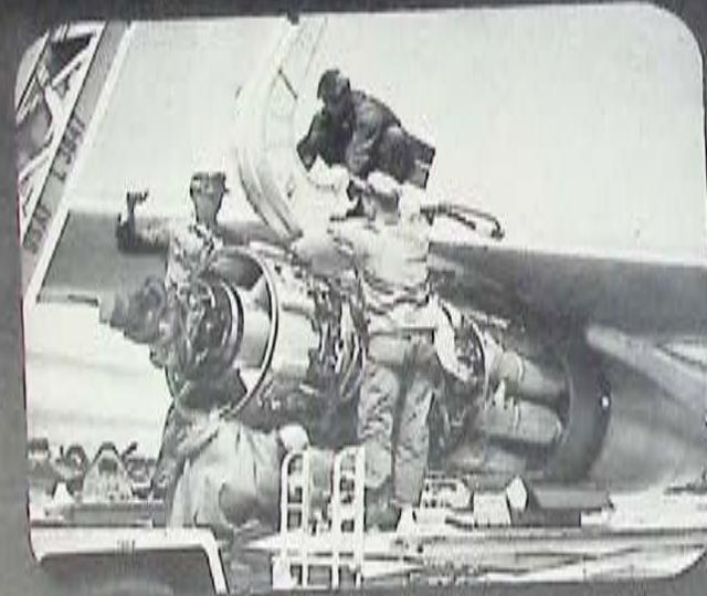
0919 New engine hoisted up while crew installs J47 fuel, oil, and electrical lines.
