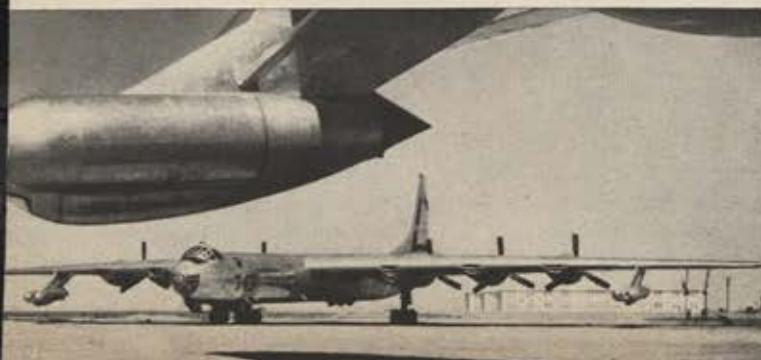
LONG J47 OPERATING TIME BETWEEN OVERHAULS is typified by B-47 No. 12234 of S.A.C. 306th Bombardment Wing. Aircraft flew more than 600 hours without a single engine change.
