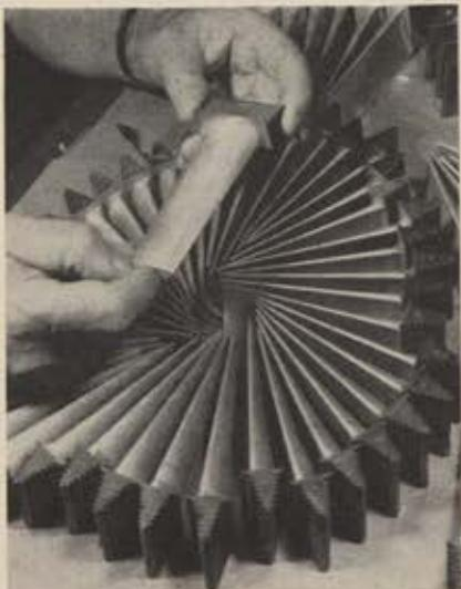
These Waspaloy turbine blades have had an acid bath to bring out grain size of each for closer inspection.
