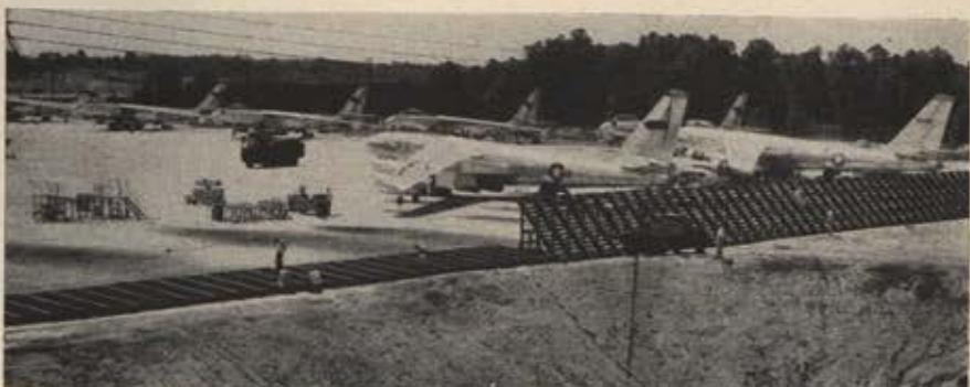
What look like bleachers on Lockheed's Georgia flight line are really jet exhaust deflectors. Steel vanes divert jet blasts and sounds into the air.
