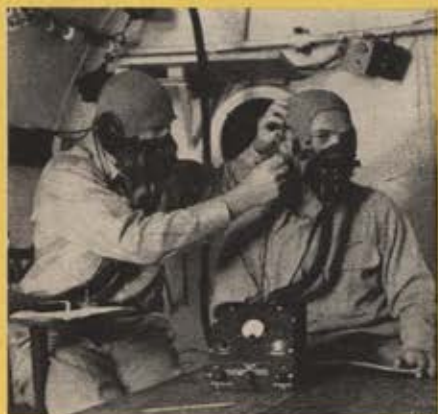
Device on ear electronically tells pilot when he's running low on oxygen. (Below) Here's an airman who gets airsick on purpose for the sake of science.
