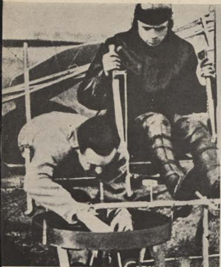
The man fumbling around in the dishpan is Riley Scott, who is about to try out his mechanical bombsight. His two 18-lb bombs hit the target, or almost, and long before the days of Norden.
