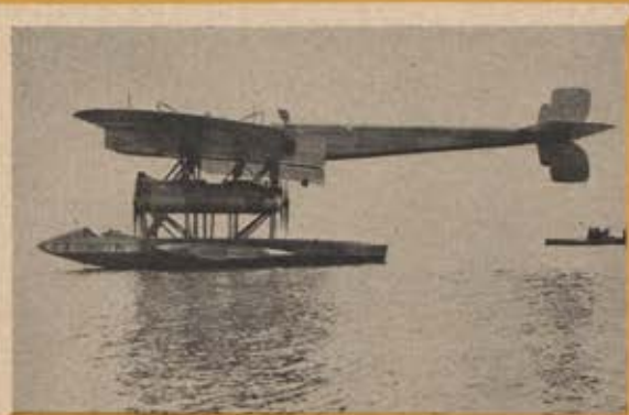
Dornier's R-4, built late in World War I, spanned 120 feet. All metal, it was powered by four 270-hp Maybachs.
