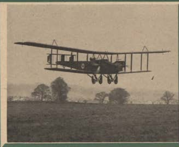
The Handley-Page was one of England's earliest giants, and the first successful Allied heavy bomber of World War I. Built in 1916, it spanned over a hundred feet. It was the first of the heavy bombers to achieve a top speed of over 100 mph. Note the thick airfoil used.
