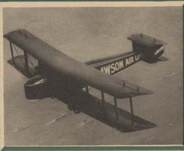
The twin-engine Lawson, completed in 1919, was the first successful luxury airliner in the U.S. Designed by Vincent Burnelli, it toured the country, trying to rouse interest in the establishment of commercial air transportation. It was succeeded by larger craft.
