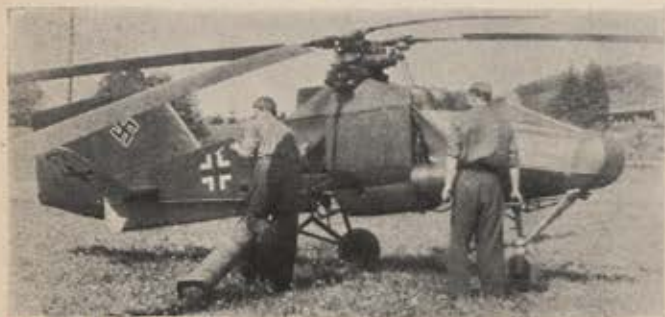
Flettner helicopter, with counter-rotating, intermeshing blades, once landed on the deck of a submarine which was moving at 18 knots.
