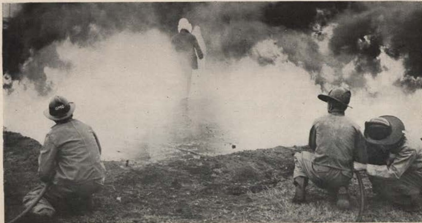
Rescuemen walk through a path cut into the flame by hosemen with fog lines. Firemen carefully hold streams low to prevent back-flashes.
