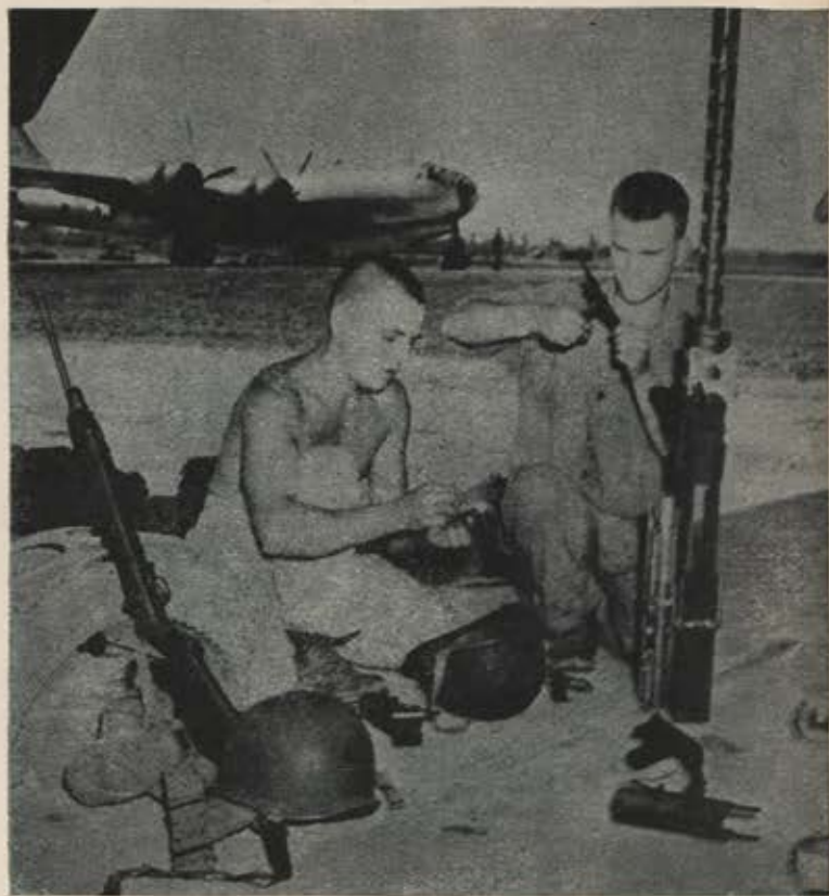
Pfc. Jimmy Carmichael and Cpl. Joe Czeremysika , armorers of the 20th Bomber Command, overhaul .50 caliber machine guns in the shade of a Superfortress at a newly constructed airbase in India.
