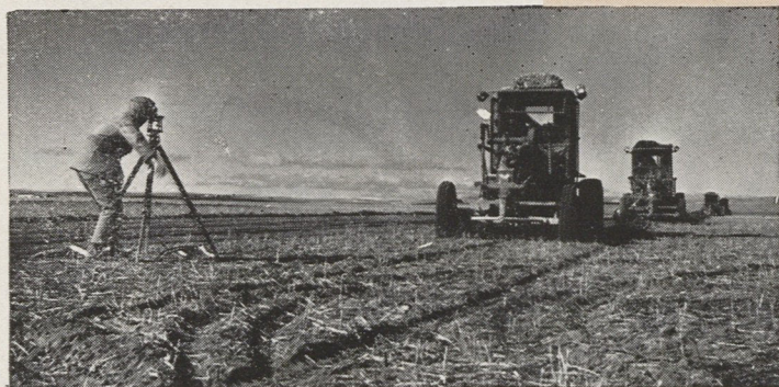
A surveyor and grading machines work simultaneously on a new airbase site.
