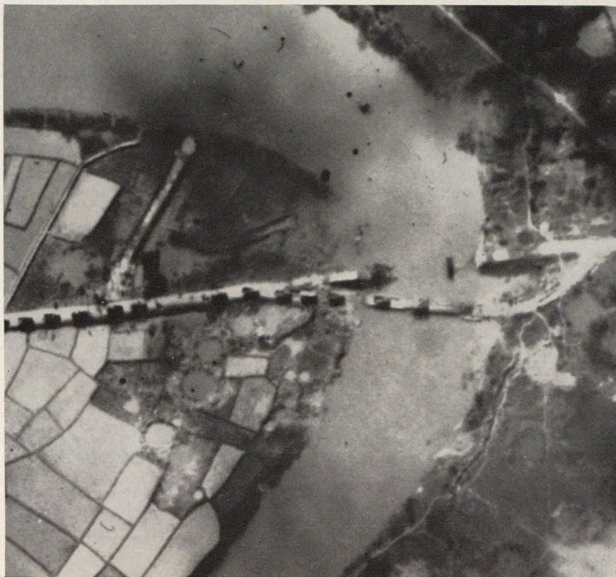
Caught in the open, a string of trucks waiting to cross a river in North Vietnam is photographed by an RF-101. The traffic jam is caused by a makeshift ferry being used to bypass a bombed-out highway bridge. The bridge was a typical choke-point target in the interdiction campaign. Since the North Vietnamese are putting great effort into building bypasses such as the one above, these targets must be hit every few days to be kept closed.
