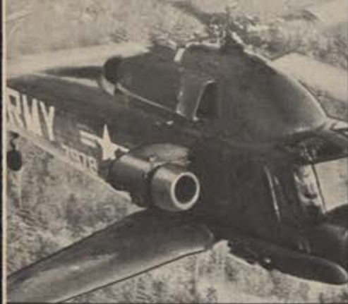
Bell X-14A deflected thrust J85 engine
