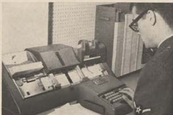
Every effort is made to verify data received from sensors around the world ranging from radars to optical telescopes. Above, information is transferred to punch cards, will be fed into Philco 2000 computer.
