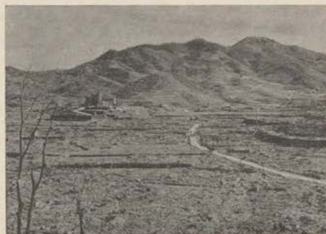
This is how Nagasaki looked after the bombing. Unlike the Hiroshima bombing, there was no fire storm at Nagasaki, and the number of casualties was about half as many as at Hiroshima. This is the residential area just east of ground zero. Catholic Cathedral ruins are in background.
