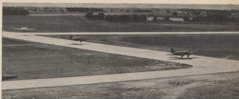
Two C-47s in tandem , with an XCG-17 (glider version of the Skymaster) towed behind them, take off in aerial version of freight train. When a safe altitude is reached, the leading plane will detach itself and return to the field for another such double-header take-off.
