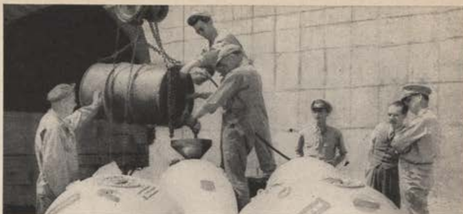
These droppable tanks with 110-gallon capacity are shown being filled with fire jelly.
