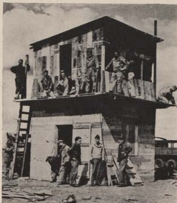
Finest materials and workmanship went into most structures at the new bases but emergency measures were sometimes required. This control tower, for instance, was built from packing cases.
