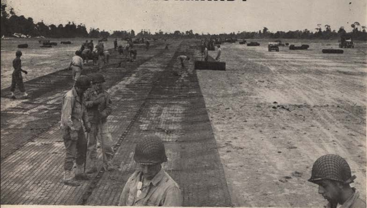
French soil gets a coating of landing mats as AAF engineers ready a Normandy landing strip for business. Note invasion-marked planes at left.
