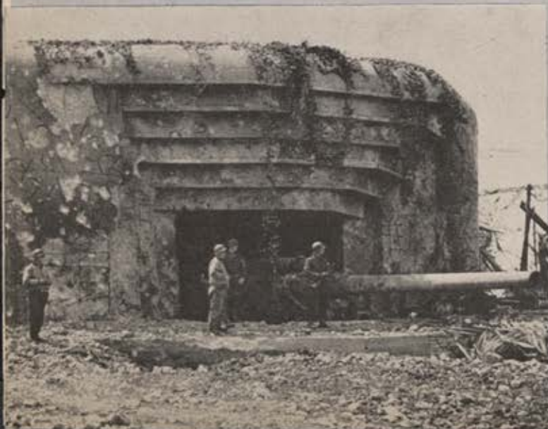
Near Quineville, France, this heavy concrete fort with its large caliber coastal gun was shattered by air force and naval bombardment.
