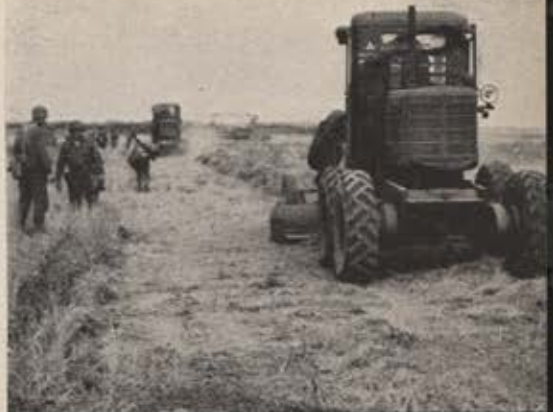
Men of 9th Engineer Command using graders.
