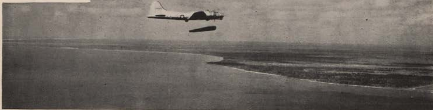
A B-17 is seen releasing the Flying Dutchman at an altitude of 800 feet. Seconds later, three huge parachutes billowed open to support the newly-developed, motorized lifeboat in its descent to the water.
