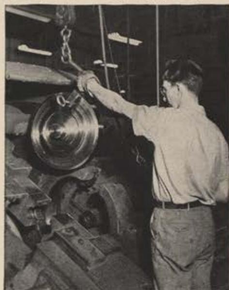
*Lowering J33 turbine wheel and shaft into special flash butt welding machine.*
