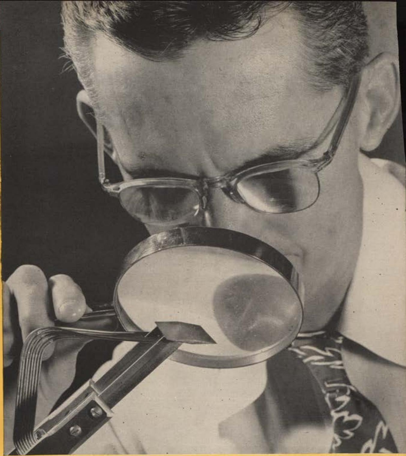
Researcher examines tiny airfoil. Each tube connects an orifice with a manometer to measure pressure.
