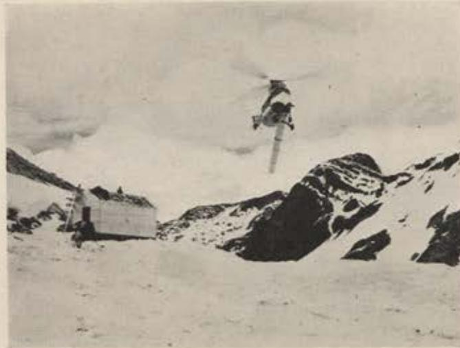
**HIGH HAUL**—In rugged British Columbia, a 50-mile power line is being built to serve an Aluminum Company of Canada plant at Kitimat. Work on this project has been enormously speeded by S-55s, flown by Okanagan Helicopters, Ltd., which can airlift almost everything needed to virtually inaccessible construction sites.
