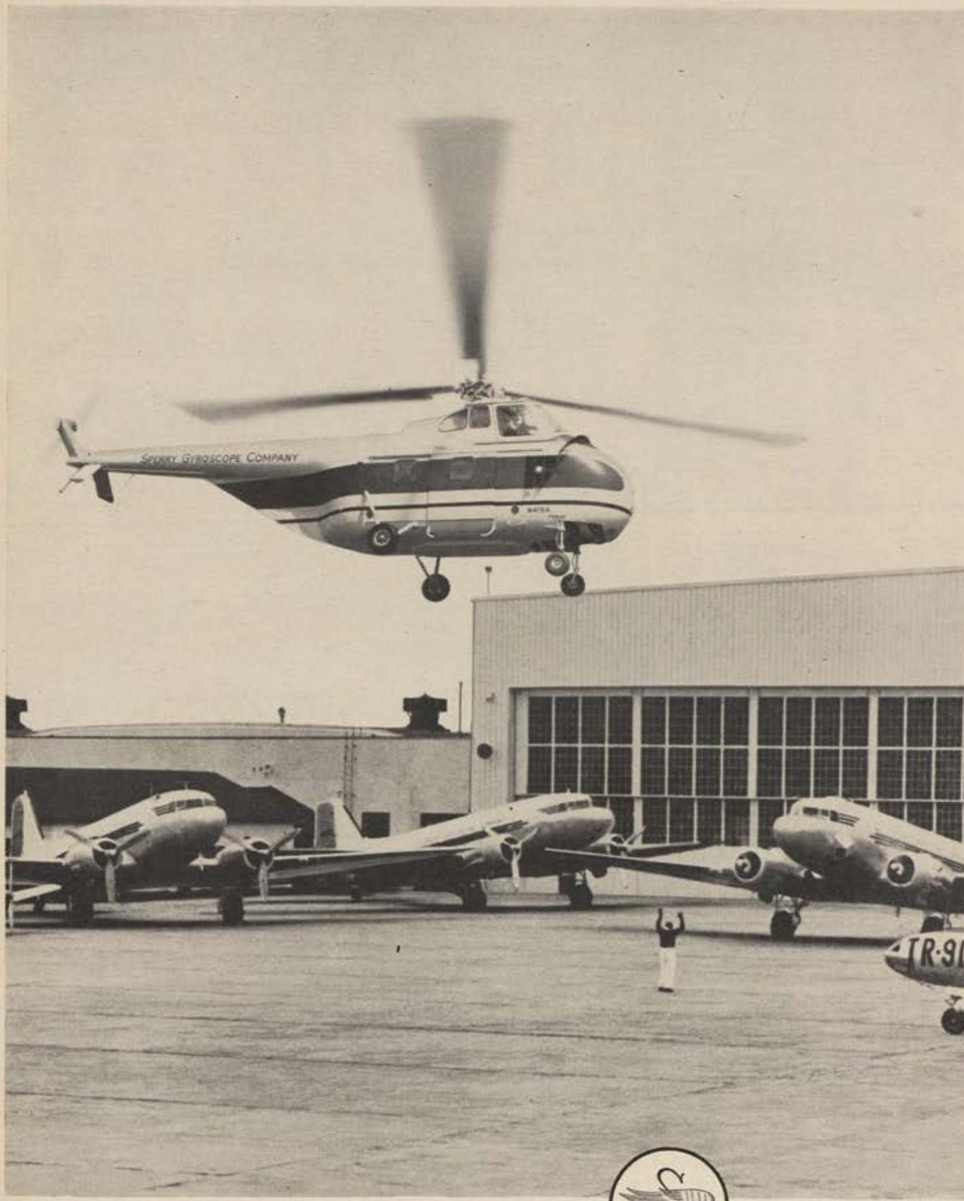
**RESEARCH TEAM-MATE**—A new Sikorsky S-55 helicopter is the latest addition to Sperry Gyroscope Company's large flight research department at MacArthur Field, Long Island. This versatile aircraft will be used as a flying laboratory, helping Sperry engineers test and develop improved instruments and other equipment for navigation and flight control.
