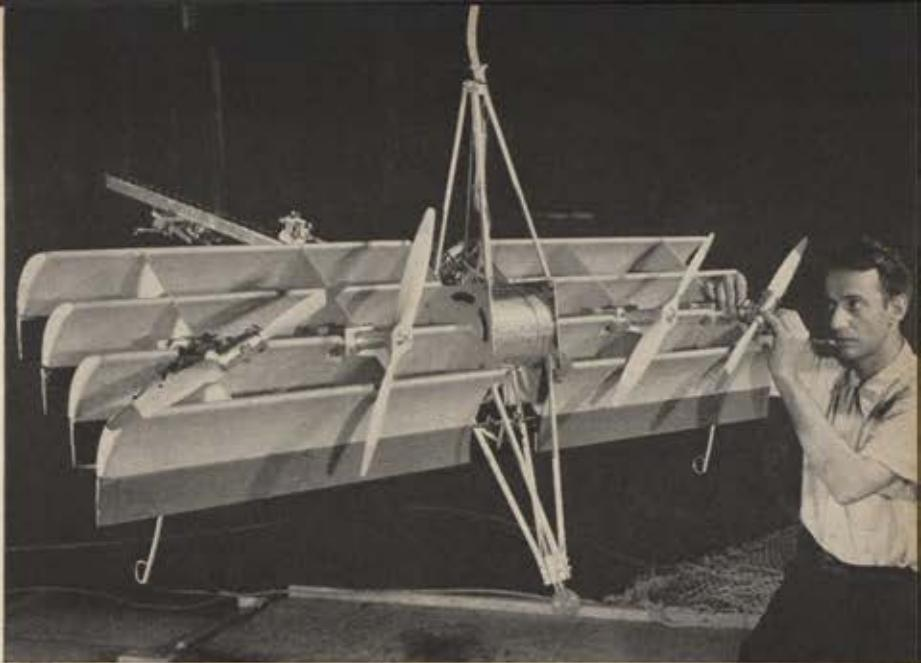
This flying venetian blind is an NACA model designed to study stability and control problems in vertical-rising aircraft. The slat arrangement deflects the slipstream downward.
