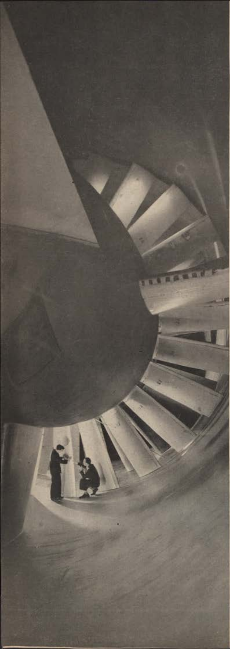
Inside the huge return passage of the NACA's 16-foot transonic tunnel, these vanes turn the airflow smoothly around a 90-degree corner. The straight bars help to reduce turbulence of the flow.
