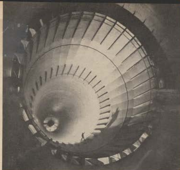
Another look at the return passage in the 16-foot tunnel. The air vents in foreground are part of an air exchange system that removes warm, slow-moving air and substitutes cool air from outside.
