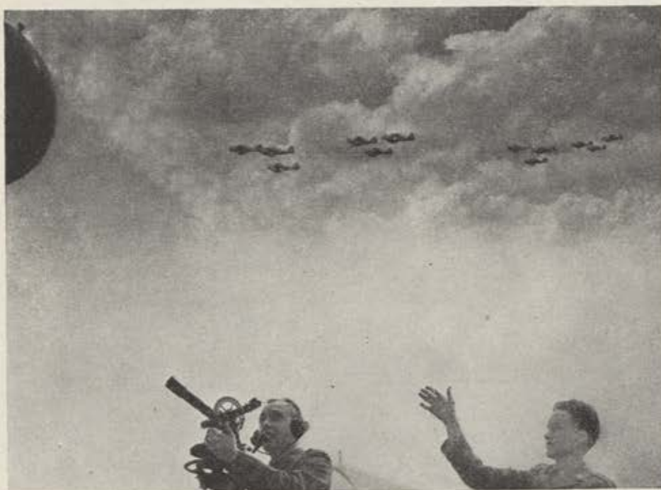
With atmospheric enemies which can be just as deadly as opposing planes and anti-aircraft fire, the airman needs to know what to expect from fog, storms, icing and headwinds. These weather men follow the pilot balloon with a theodolite to learn the speed and direction of wind aloft.
