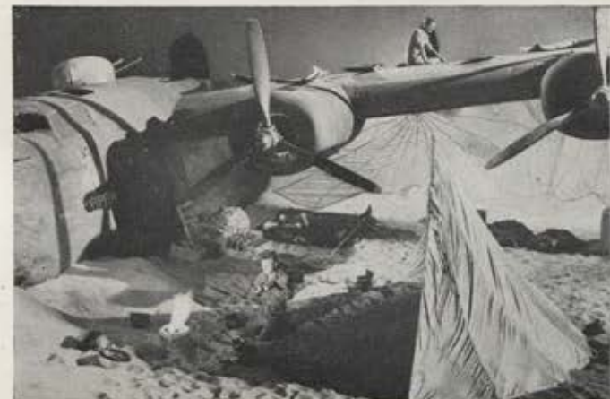
Plane's equipment is utilized to aid the crew's fight for survival. Ship's toilet is converted into a stove by filling it with sand and gasoline. Parachutes become awnings against the burning desert sun. Wings are scraped so sun's reflection may attract a rescue plane.
