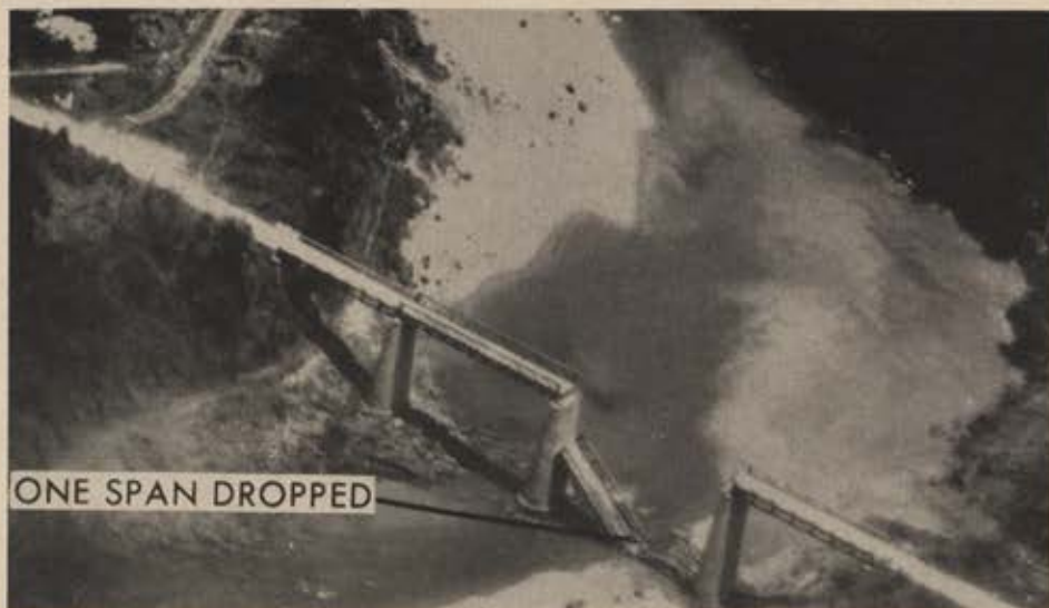
Prime targets in escalation of air war in Vietnam in recent weeks have been supply lines. One of the spans of this 350-foot highway bridge along Route 12 was completely destroyed in a mid-April US raid.
