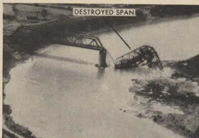
This was a two-span steel truss railroad bridge in North Vietnam before it was visited by US airpower in early April. One span of the 330-foot-long structure was completely destroyed and fell into river. Approaches were damaged too.
