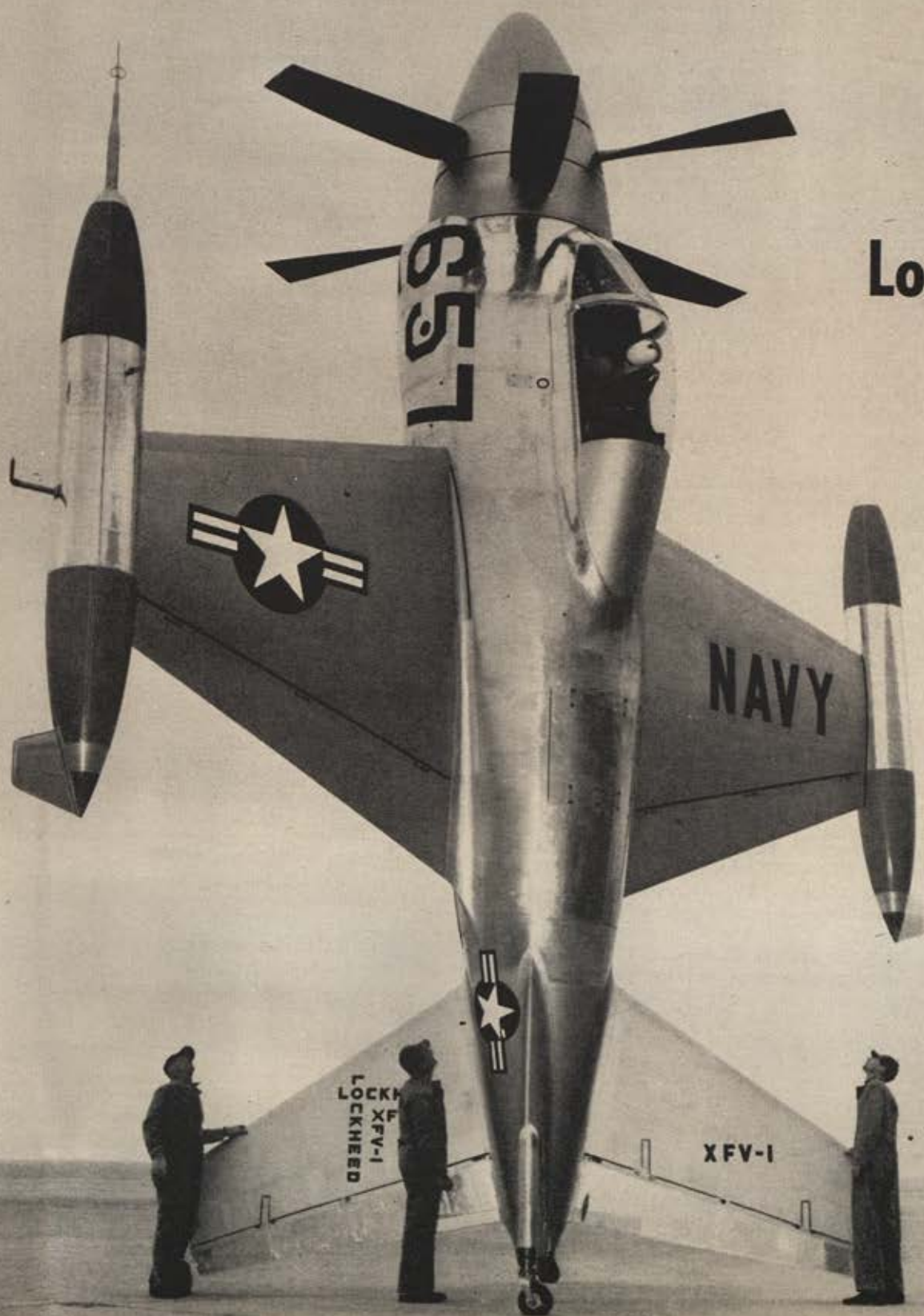
SPECIAL CRADLE LIFTS XFV-1 from prone position (for servicing) to upright for vertical takeoff.
