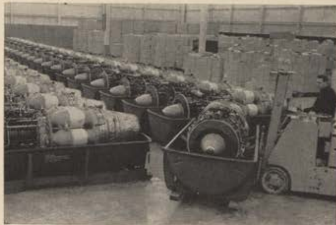
In its plant near Toronto, Avro is also building Orenda turbojets that power the CF-100 and Canadian-built F-86s.
