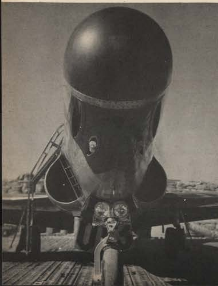
Eye of the night. Housed in the bulbous nose of the F-94 is the radar set that searches the night and fingers out enemy night fighters bent on destroying USAF bombers. The Starfire's afterburner gives additional thrust on take-off and makes possible speedier interception of "bandits."
