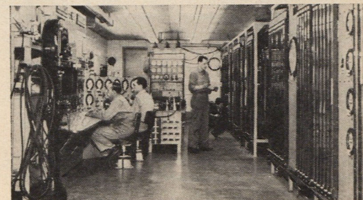
Test cell control room is "floated" on rubber cushions and suspended in air to insure instrument accuracy.
