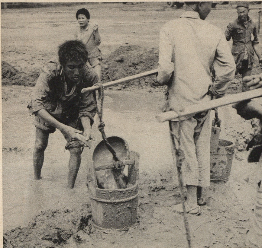
Hundreds of thousands of workers using primitive methods and substituting mud and clay for cement constructed the B-29 runways in China. Without modern machinery to work with, these coolies did a remarkably competent job.
