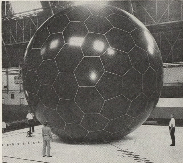
New type of communications satellite scheduled for launch by U.S. Air Force in July is this 30-foot-diameter (9.1 m) sphere developed by Goodyear Tire & Rubber Co. After being inflated in space, balloon's skin will photolyze, or disappear, with wire grid remaining rigid to reflect radio waves.
