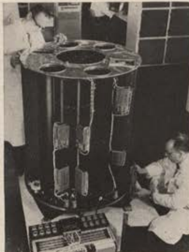
Cook Electric Co. scientists assemble University of Wisconsin Experiment Package, containing telescopic and spectroscopic equipment, similar to the one which will be carried aboard the first Orbiting Astronomical Observatory.
