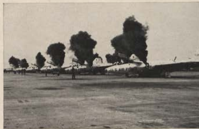
Clouds of black smoke are produced by explosive cartridges used to start B-57 engines. Canberras, formerly based in Japan, were destined for ANG when rerouted to Vietnam.
