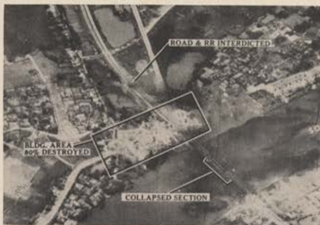
This is what the railroad and high bridge at Dong Phuong Thuong in North Vietnam looked like after getting a taste of airpower as the air war was stepped up. Post-strike reconnaissance photographs show the extensive bomb damage.
