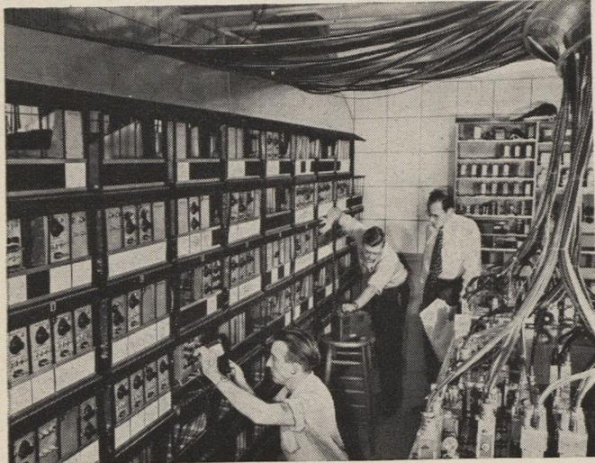
**COMPUTER.** Important to guided missile research is this electro-mechanical analogue computer designed by Boeing engineers. Simulating missile flight, the computer saves months of time and countless dollars otherwise spent in experimental test firing.
