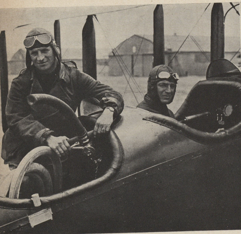
History's first air-to-air refueling. Left, just before takeoff, Lt. Frank Seifert holds the nozzle of the hose while Lt. Virgil Hines, who flew the DH-4B refueling plane sits in front cockpit. Right, the operation itself, June 1923.
