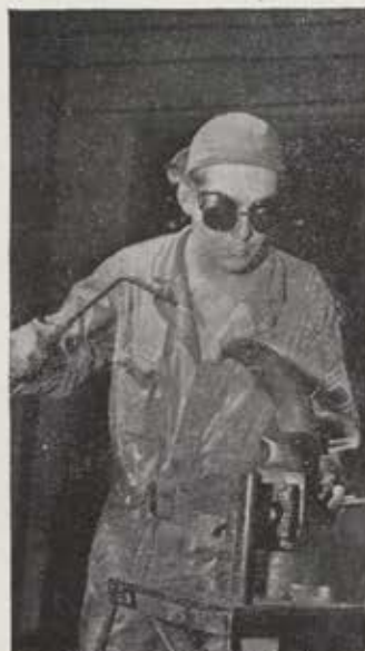
From the pattern supplied by a broken bakelite cannon plug (upper left) the sergeant made the substitute (below). He is shown testing the buffalo horn with a blow torch to determine the heat resistance.
