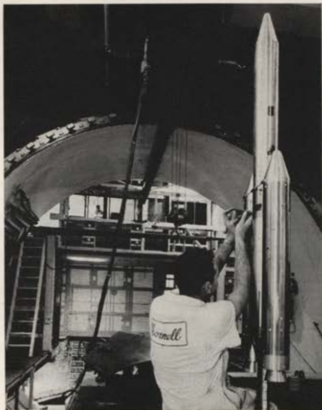
Large wind-tunnel model of the Titan III-C is readied for testing in transonic tunnel at Cornell Aeronautical Laboratory (below). Assembly and checkout of Titan III booster will take place in a building 215 feet high at Cape Canaveral (sketch above). Little checkout will be needed on the pad.
