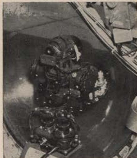
Interior sighting station at blister of a B-29—one of five such gunnery positions coordinated by central fire control system.
