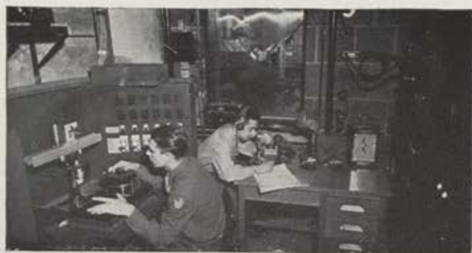
The enlisted man with earphones is talking to the man inside chamber and observing his reactions to sub-zero temperatures while operating a machine gun. Thermometer showed forty below zero when picture was made.
