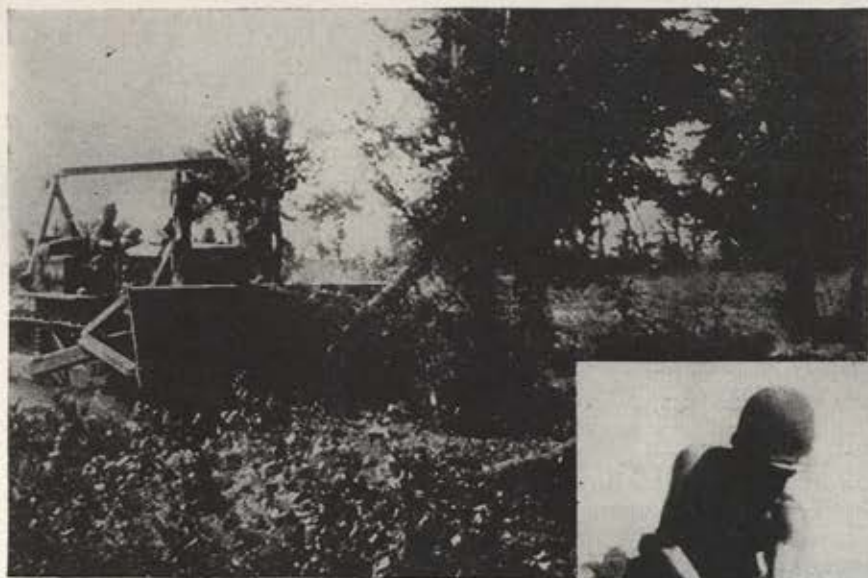
Establishment of airfields was of first importance. Just one mile from the beach aviation engineers selected two adjoining farms for conversion into an emergency landing field. Trees were bulldozed and a fast job with pick axes helped level off the new runway. First to use the field were two P-38s which came in exactly 24 hours after the cotton and wheat fields were taken over by aviation engineers. The task of engineers in advancing our airbases closer to the enemy and his supplies is vital in maintaining control of the battle sky.
