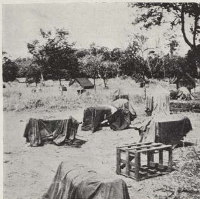
An excellent job of garnishing is being done on this drape job over an operations tent of a heavy bombardment group. The net has been spread so that outlines are vague when seen from the air and the garnish has been dyed to blend well with the terrain. No telltale shadows are cast.
