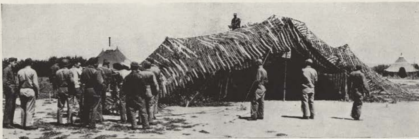
An excellent job of garnishing is being done on this drape job over an operations tent of a heavy bombardment group. The net has been spread so that outlines are vague when seen from the air and the garnish has been dyed to blend well with the terrain. No telltale shadows are cast.
