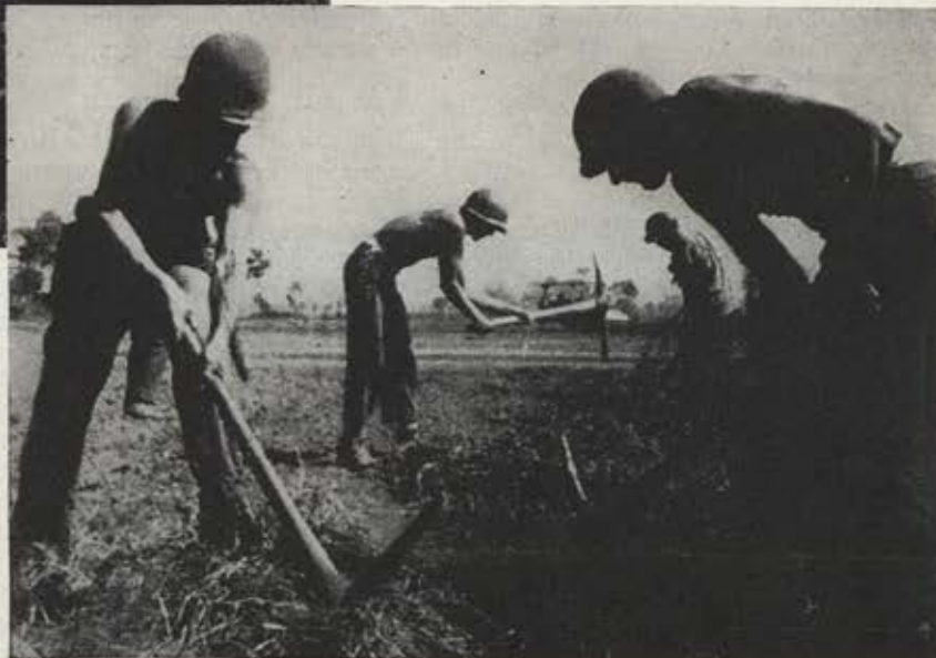
Establishment of airfields was of first importance. Just one mile from the beach aviation engineers selected two adjoining farms for conversion into an emergency landing field. Trees were bulldozed and a fast job with pick axes helped level off the new runway. First to use the field were two P-38s which came in exactly 24 hours after the cotton and wheat fields were taken over by aviation engineers. The task of engineers in advancing our airbases closer to the enemy and his supplies is vital in maintaining control of the battle sky.
