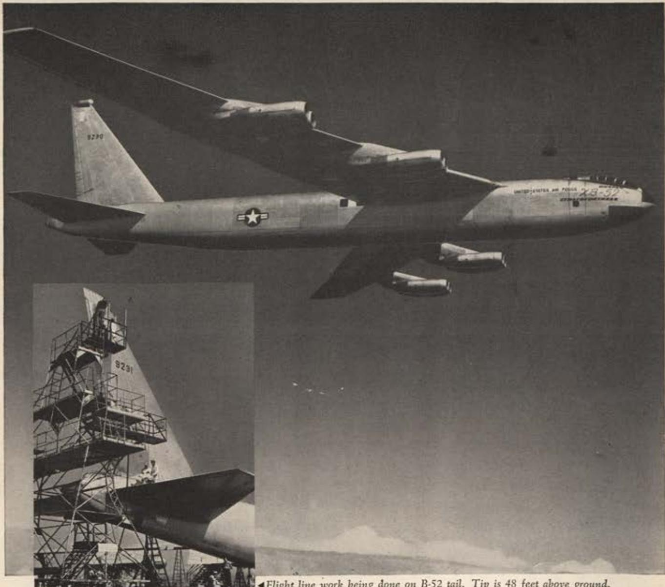
◀Flight line work being done on B-52 tail. Tip is 48 feet above ground.
