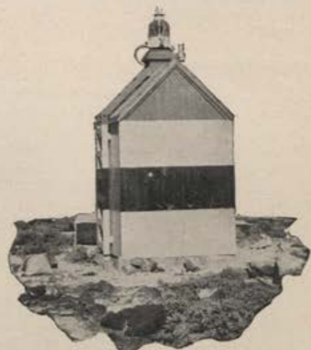
Long-term beacon light is automatically controlled. Shack contains acetylene tanks to fuel lantern nightly for an entire year.
