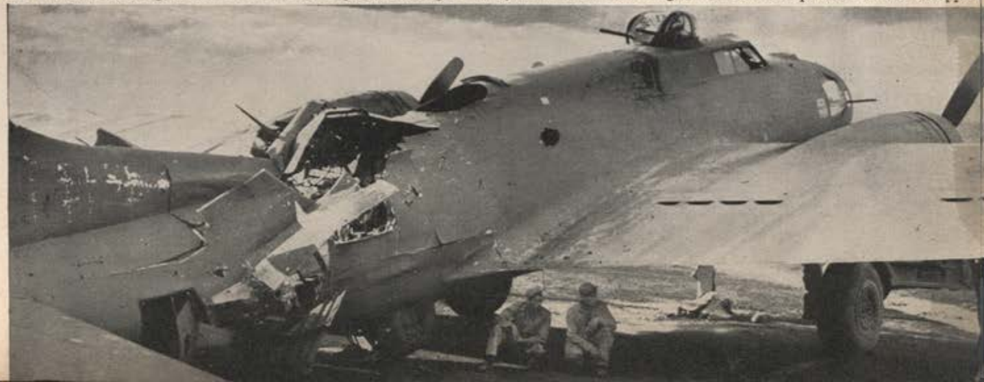
Riddled with flak holes sustained on a mission over Debreczen, Hungary, this B-17 almost split in two when its tail wheel gave way during landing. No one was hurt. Test flights show B-17s have enough extra strength to carry bombs under each wing and this bonus helps when bomber is crippled.
