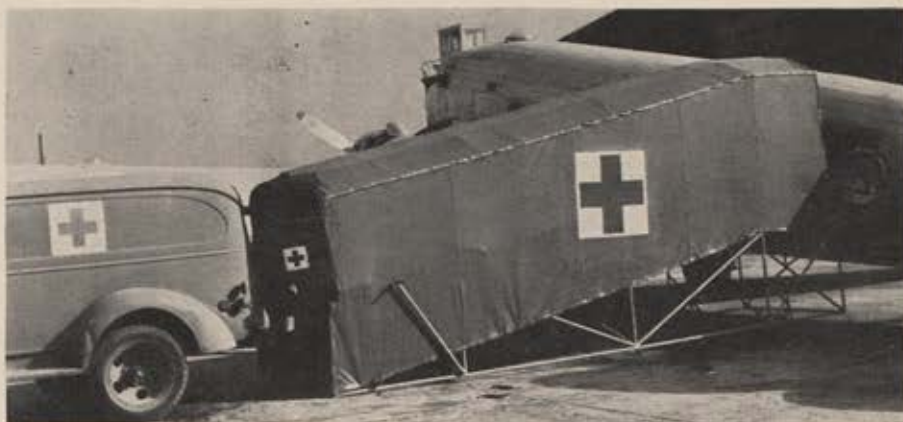
Unloading of patients from C-47 hospital plane into waiting ambulance is made easy by means of this canopied ramp constructed from salvage by the 20th Ferrying Group, Nashville.
