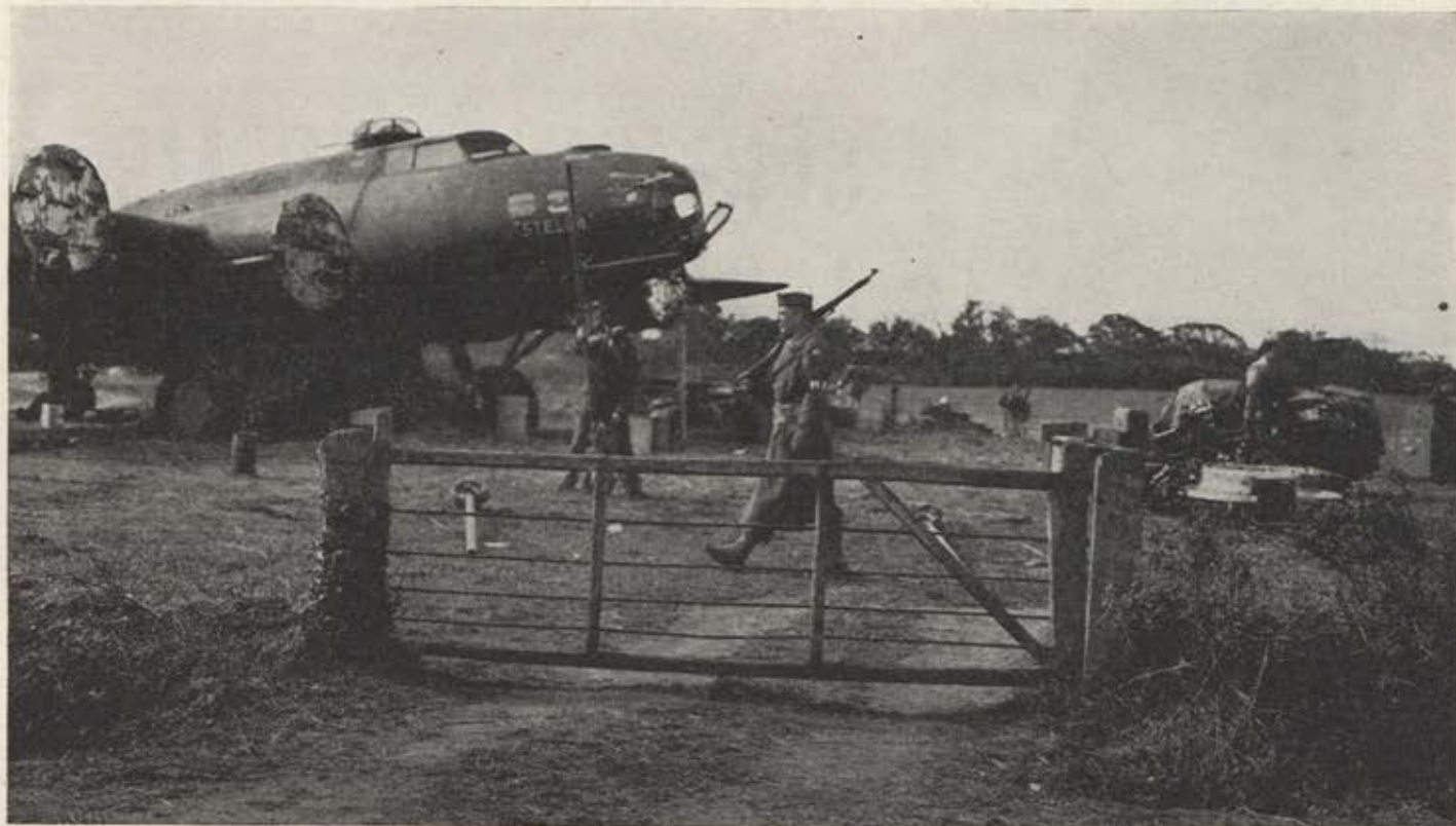
Mobile repair units for crashed aircraft, like medical units for injured personnel, follow their planes and make emergency repairs. The 8th Air Service Command maintains units which travel wherever disabled planes have landed. This plane's four engines and ball-turret were damaged in an emergency landing, but the bomber was able to take off from a make-shift runway after the mobile unit had completed the repair job.
