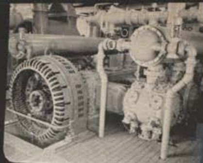
Compressor delivers up to 200 lbs. pressure per square inch.
