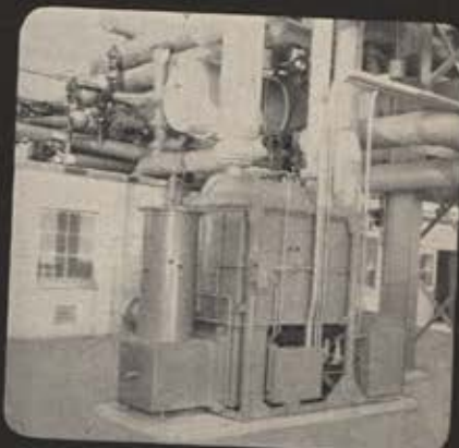
Air heater produces temperatures ranging up to 800^{\circ}\text{F} .
