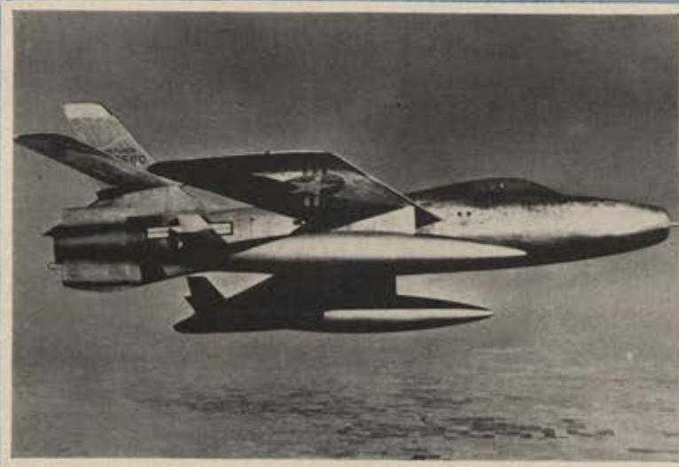
Republic also made news with its XF-91, an American experimental aircraft incorporating the characteristics of a combat-type fighter, which made its first faster-than-sound flight at Edwards AFB. The XF-91 is equipped with a GE J-47 turbo-jet delivering 5,200 pounds thrust plus afterburner, and also a 6,000-lb.-thrust Reaction Motors rocket engine.
