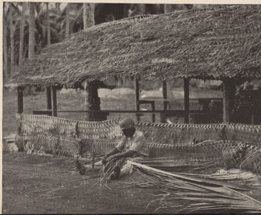
A butcher knife snitched from the mess hall helps this colored soldier expertly weave the walls of a new building from palm fronds.
