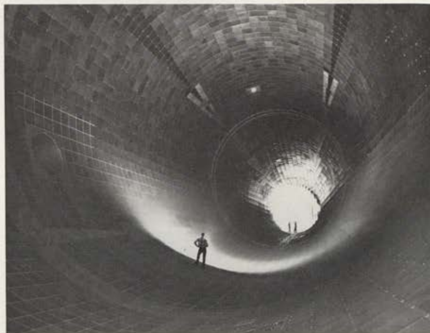
This supersonic wind tunnel can handle 650° F airflow required to simulate flight at velocities up to Mach 4 in its 16-foot (4.8 m) test section. The largest of its type in the world, the tunnel is located at the U.S. Air Force's Arnold Engineering Development Center in middle Tennessee. Above, technician checks the circuit's interior, lined with stainless steel insulated panels to handle the tremendous airflow at very high temperatures.
