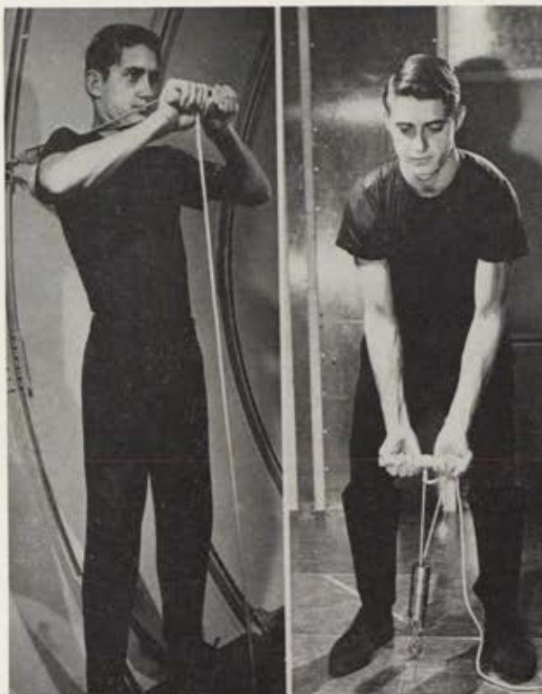
This Exer-Genie exercise device, shown being demonstrated in Lockheed Missiles & Space Company's space chamber at Sunnyvale, California, could help astronauts keep in good physical condition in the weightlessness of space. The device consists of a small metal cylinder through which a nylon line is pulled. The force required to pull the line through the cylinder can be varied.
