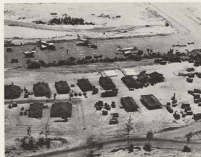
Air view of Chu Lai shows A-4 maintenance being conducted out of doors. Tail section of the aircraft at upper left has been removed, exposing the engine. Marines are encamped in tents.
