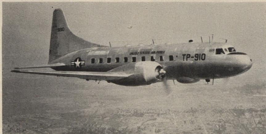
First flight picture of the Air Force's new T-29 navigational trainer, built by Consolidated Vultee is shown here. The high-speed ship, which resembles the airline's Convair Liner, is the first plane designed especially to train navigators in groups. Four astrodomes on top of the fuselage are provided for 14 students and instructors. Some of planes' 18 antennas are visible here.
