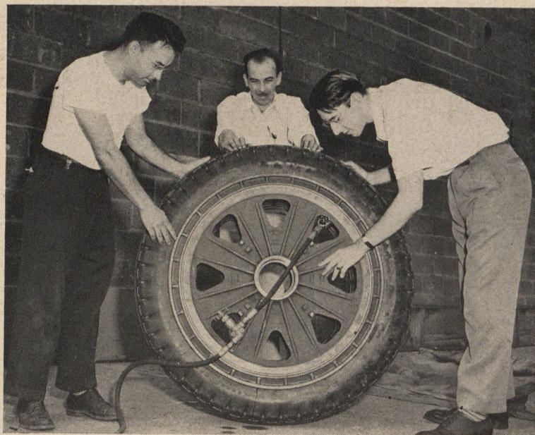
Before and after fotos of Northrop XF-89 wheel assembly subjected to a static "burst" test by Goodyear Rubber Co. Unit blew apart
